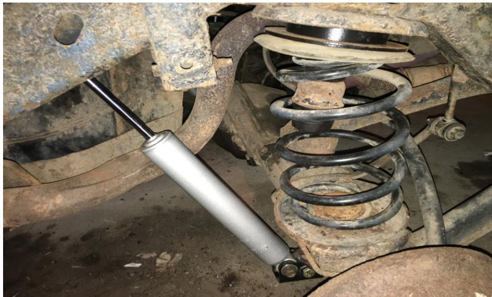
Finished installation with new shock, shock bracket and spacer.
