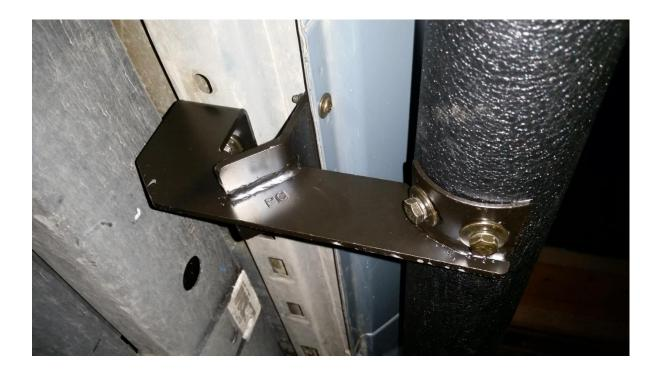
8.) Refer back to step 3 and finish tightening up all loosely installed hardware. Then continue to tighten all loosely installed hardware in steps 4 and 7.
