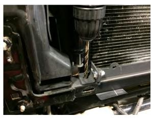
Step 5: With the brackets centered on the radiator support, mark the location and drill a 9/32" hole through the lower radiator support.
