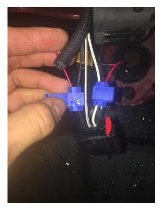
15. Again, push down on the metal piece with the pliers and close the tap connector top.
