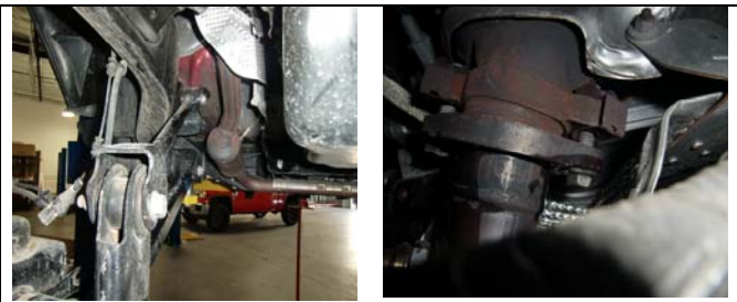
17. Unbolt the passenger side upper arm and install the new arm. You may need to flex the exhaust to remove the upper arm bolt. Tighten the upper arms on both sides. Then reinstall the bolts for the exhaust.
