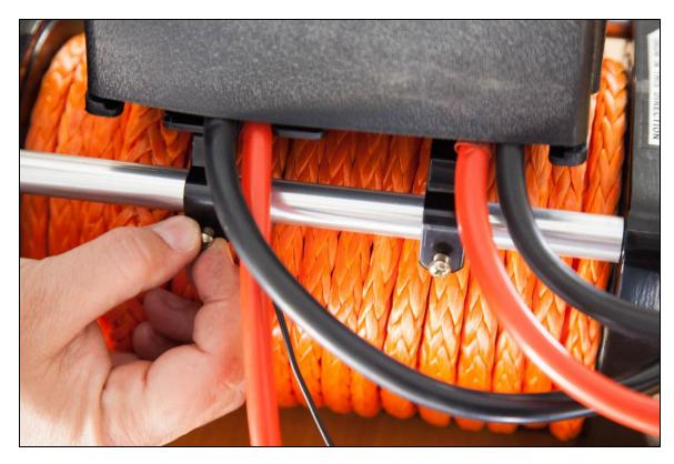
13. Rotate winch assembly forward until ground wire mounting bolt is visible. Remove ground wire mounting bolt, split washer, and flat washer.
