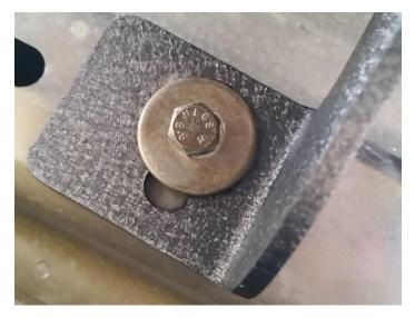
Note: Make sure that the "I" bracket is on the inside of the pinch seam.
