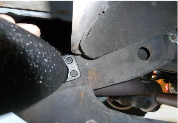
3. With guard in final mounting position, mark the frame using the mounting holes in the guard as a template. *Be careful not to move guard while marking holes.*
