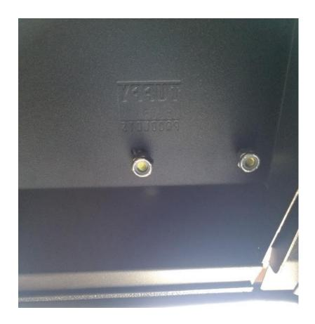
6. Repeat for all other modular gear anchors in the chosen configuration. The final product should look like this, depending on the chosen configuration and placement. Be sure to vacuum all metal shards on top of and under the installation points.
