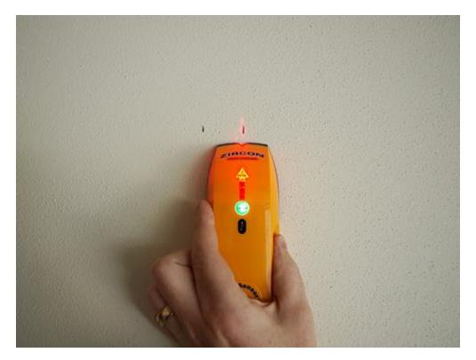
2. Begin by installing the left Lower Bracket of the Freedom Mount. Determine the height you wish to place the Lower Brackets before drilling pilot holes. The placement of the Lower Brackets will be based on one's personal preference of the location where the Freedom Panels will be stored. **Note:** Bolt holes need to be drilled at least 2" into the stud past the drywall.
