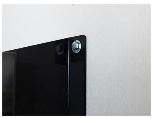
4. Place a level on the Lower Bracket to help determine the location of the second pilot hole. With the second pilot hole drilled, place a washer on a lag bolt. Insert the lag bolt through the Lower Bracket hole and into the wall. Tighten both lag bolts securing the bracket to the wall.
