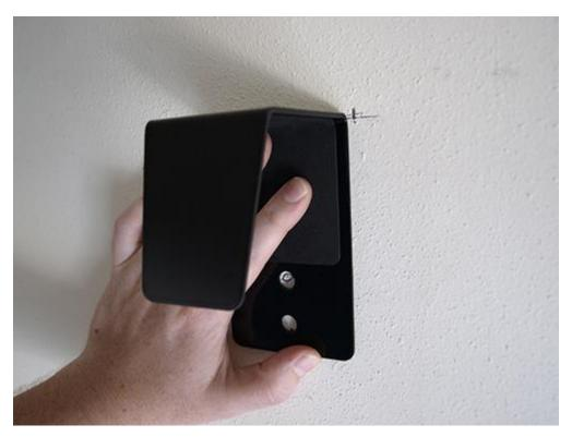
7. With the Retainer Bracket level, drill a pilot hole into the wall through the bottom hole of the Retainer Bracket. Place a washer on a lag bolt. Insert the lag bolt through the Retainer Bracket and into the wall. Tighten both lag bolts securing the bracket to the wall.
