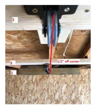
4. For Parallel ceiling joist configuration the mounting locations will be the same for all 3 of the pulleys, but pulleys 1, 2 & 3 referenced above will be attached to a single longer 2x6 mounted to the ceiling joists. Make sure to select a length that is at least long enough to span several ceiling joists while still allowing for a spacing of 32" between pulleys 2 & 3 and making sure that pulley 3 is ½" left of center. See diagram below.
