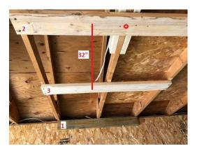
2. Mount the dual pulley in the center of the 2x6 (number 1 in the photo above) using the supplied screws (4). Next mount a single pulley in the center of the 2x6 (number 2 in the photo above) using supplied screws (4).
