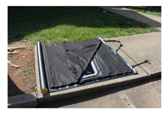
13. With windows in place and all layers of protective cloth covering the plastic roll tube toward straps. It is not necessary roll really tight but let the tube do the work for you. Smooth the fabrics layers as you roll.
